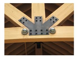
Exposed truss ends require immediate caulking and painting. See photo with camera location.
